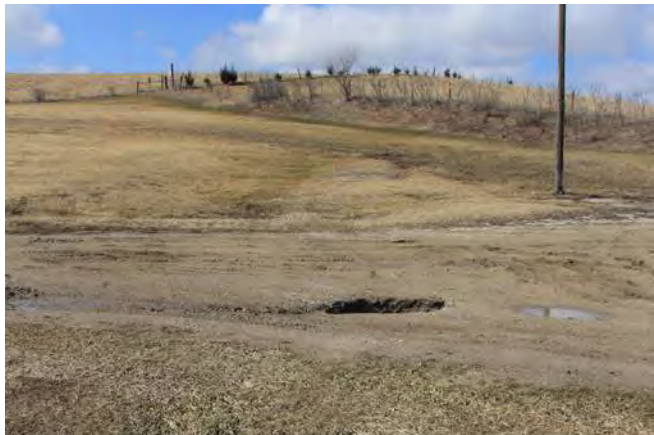
Severe erosion on the gravel road. Looking North.
