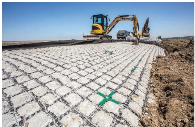
For I-680 "betterments" to add resiliency to the slope of the roadway include the installation of concrete flexamat.
