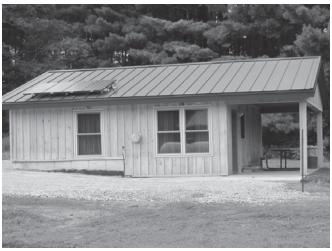
An exterior view of a cabin shows the solar panel, steel roof, and exterior siding from wood harvested in a county forest (landscaping yet to be completed).
