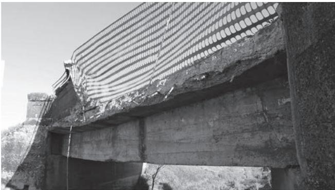
This 100 year-old concrete drainage structure has experienced considerable deterioration and has been repaired after recent high water storm event causing undermining of the foundation. The additional road use tax in 2015 has allowed adding this structure to our construction program for 2016.
