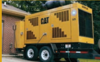
Permanent or portable generators
