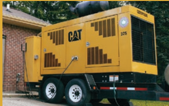
Permanent or portable generators
