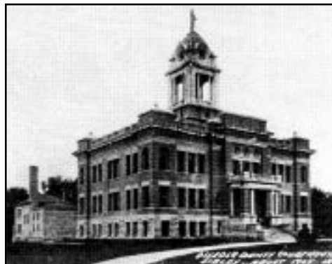
Left: Osceola County Courthouse as it appeared in 1902. Below: The current Osceola County Courthouse in Sibley, IA.
