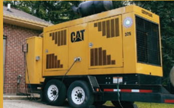
Permanent or portable generators
