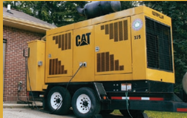
Permanent or portable generators
